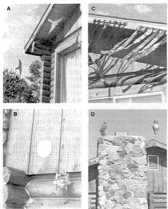
Figure 1: Hawk mobiles (A), 7<sup>1</sup>/<sub>2</sub>-inch diameter shaving mirrors and pinwheel (B), black plastic or aluminum foil strips (C), and owl effigies (D) can be mounted near damage sites to frighten woodpeckers.
