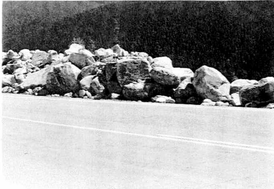
Photo 3 - Typical rocks removed from work zones during scaling operation.
