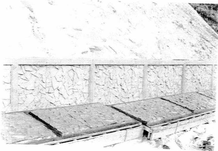
Photo 9 - Finished concrete wall after removal of random stone forms.
