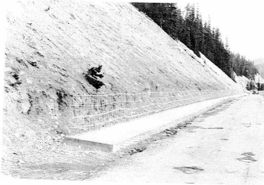
Photo 8 - Concrete wall construction .
