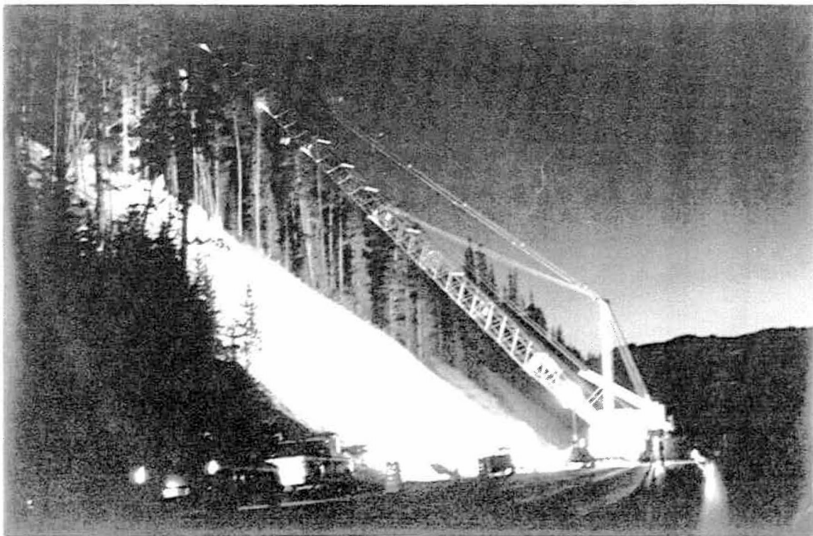
Photo 7 - Nighttime scaling operation being performed in work zone 3 using a crane.
