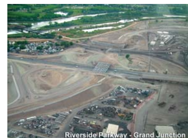
Riverside Parkway - Grand Junction
