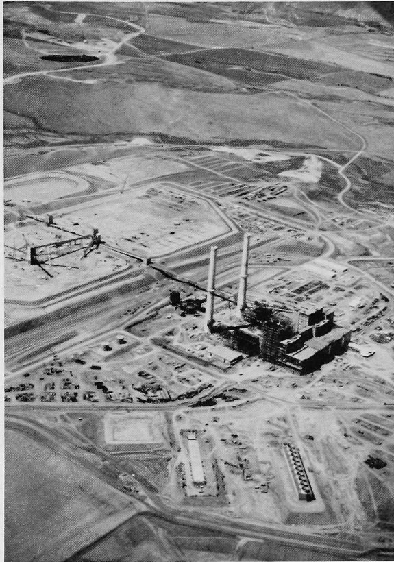
Figure B1. Coal fired power plant at Craig, Colorado.
