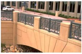
Lower Parapet with Open Railing Above
