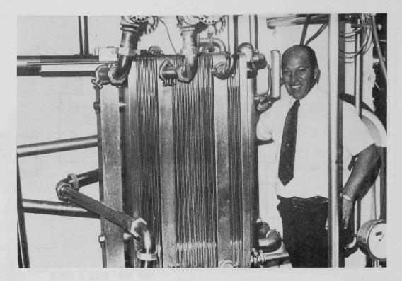
Figure 14. Heat Exchanger for Milk Pasteurization at Medo-Bell Dairy, Klamath Falls, Oregon.
