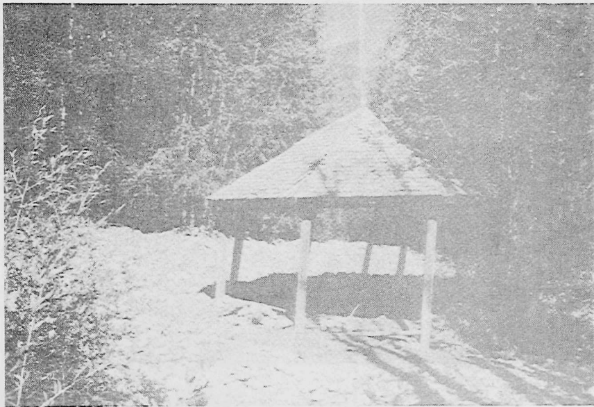
Figure 9. Top of park bandstand in town of Marble, lower part was buried by coarse mudflow debris of 1945 mudflood on Carbonate Creek.
