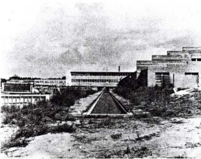
Fig. 3.4. Current meter tow tank. Dimensions of the tank are: Length - 200 ft; width - 5 ft; depth - 5 ft.
