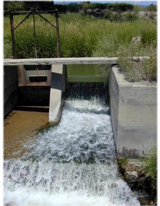
Figure 13: Sluice Gate for Flow Control
