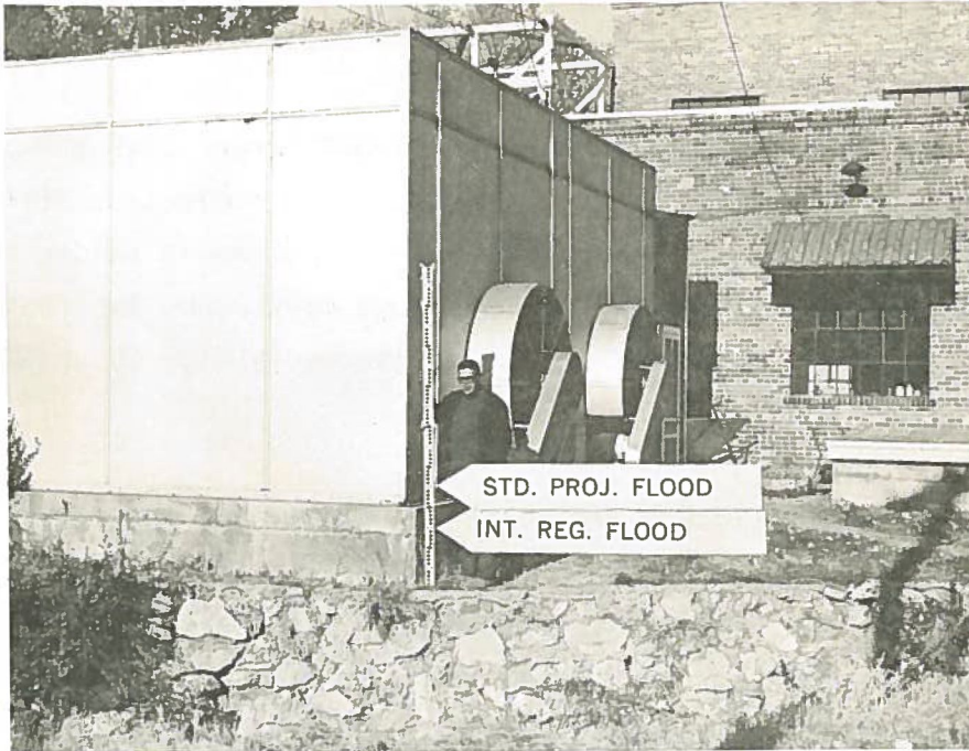
Fig. 5. City power facilities located just upstream of the Chicago, Burlington & Quincy Railroad bridge.
