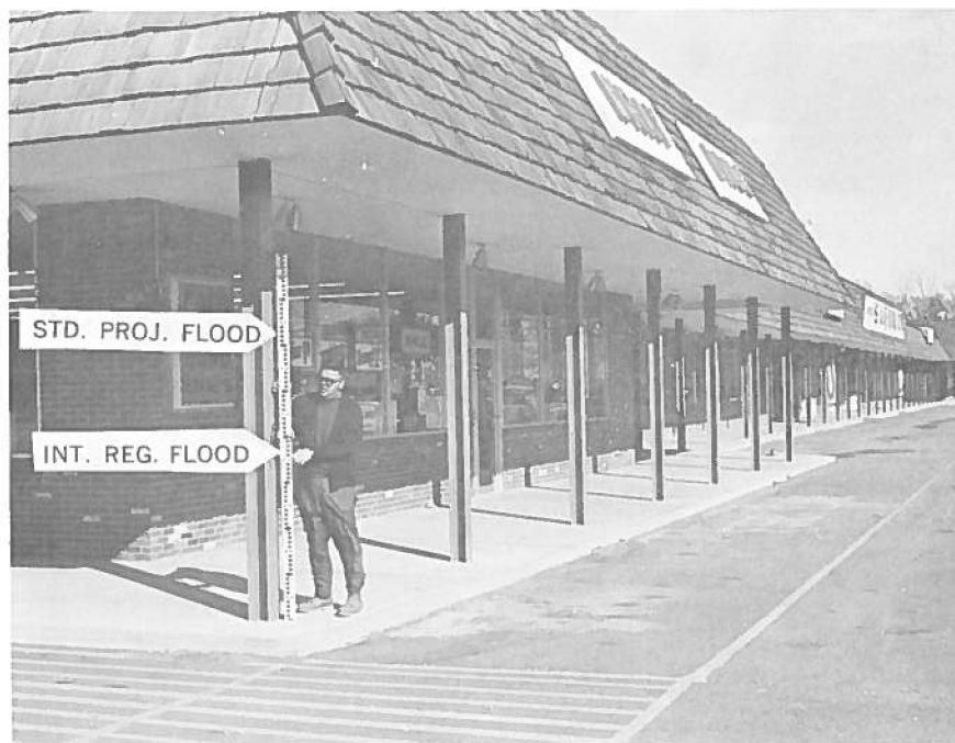
Fig. 12. Southwest corner of shopping center shown above.
