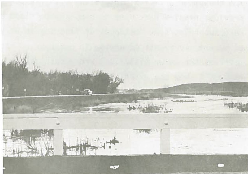
Fig. 2. May 1958 flood. Floodwaters upstream of the U. S. Highway 385 bridge.
