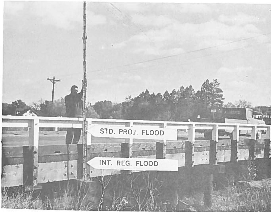
Fig. 13. Upstream side of U.S. Highway 385 bridge at Wray.
