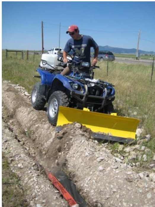
Figure 4.6: The installation of the Senstar Perimitrax® cable. Filling up the trench (Photo: Marcel Huijser, WTI/MSU).
