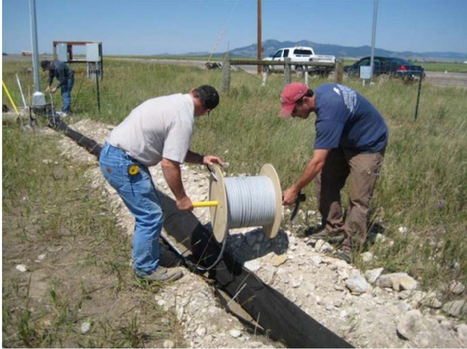
Figure 4.5: The installation of the Senstar Perimitrax® cable. The cable is embedded with sand and wrapped in geotextile (Photo: Marcel Huijser, WTI/MSU).
