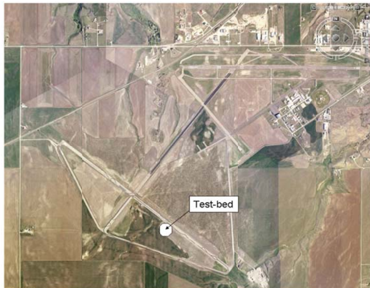
Figure 4.1: The location of the test-bed along a former runway at the Lewistown Airport in central Montana, USA. The current municipal airport is located on the upper right of the photo.
