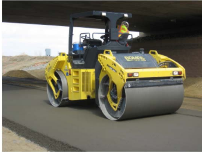
Fig. 1.7 RCC pavement is compacted by a vibratory roller
