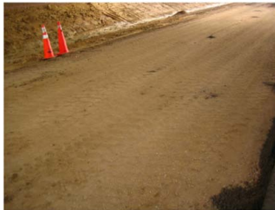
Fig. 1.1 The base course is prepared before placing RCC mix
