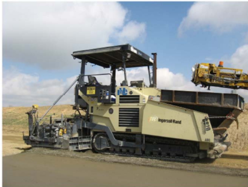
Fig. 1.6 RCC is placed using a Titan paver
