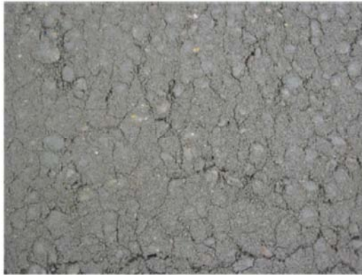
Fig. A.2 Surface texture of RCC pavement
