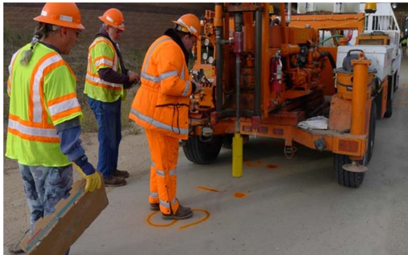
Fig. 3.19 Preparation for taking concrete samples from the traffic lane at WCR 28
