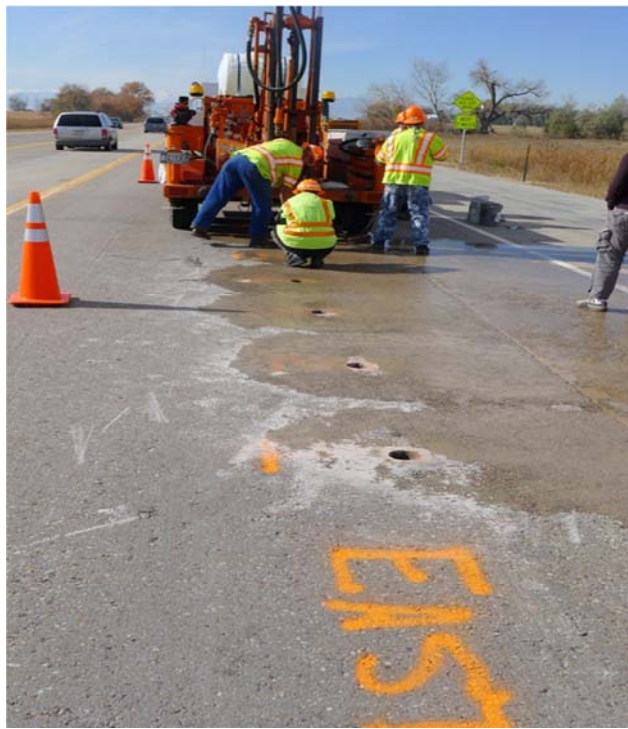
Fig. 3.21 Extracting concrete samples at EB 66
