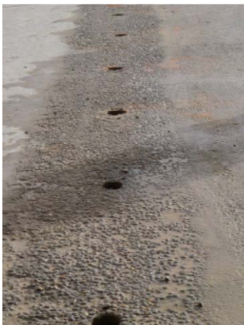
Fig. 3.4 Concrete cores are taken from the longitudinal middle strip at WCR 28
