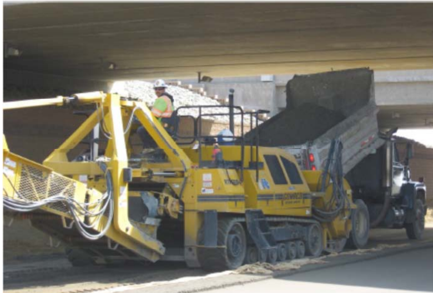
Fig. 1.4 RCC mix is transported to a paver by a dump truck
