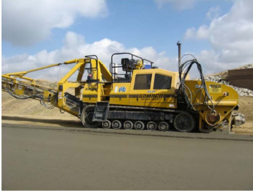
Fig. 1.5 RCC mix is transferred to the paver using a GOMACO RTP-500
