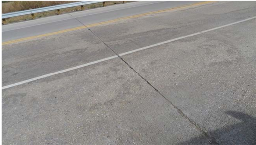
Fig. 3.14 A saw cut joint in the pavement at EB 66
