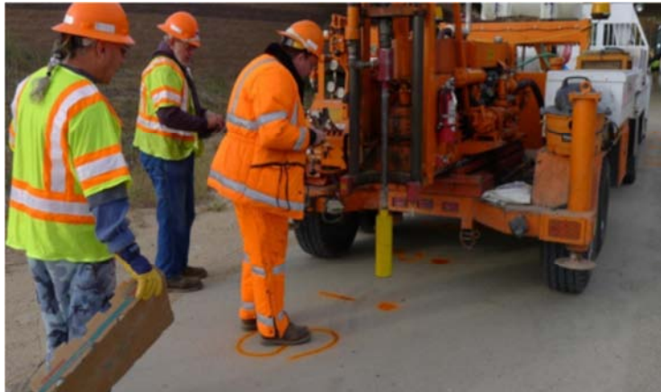
Fig. 3.3 Coring in-lane concrete samples at WCR 28
