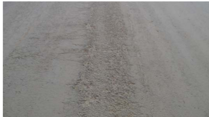
Fig. 3.2 Surface texture in the longitudinal direction in the middle strip at WCR 28
