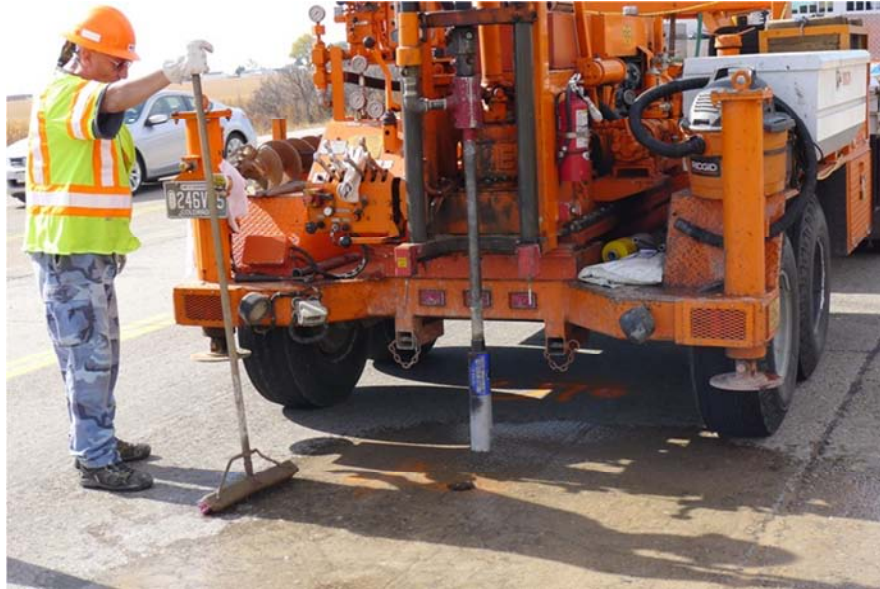
Fig. 3.22 Extracting concrete samples at WB 66
