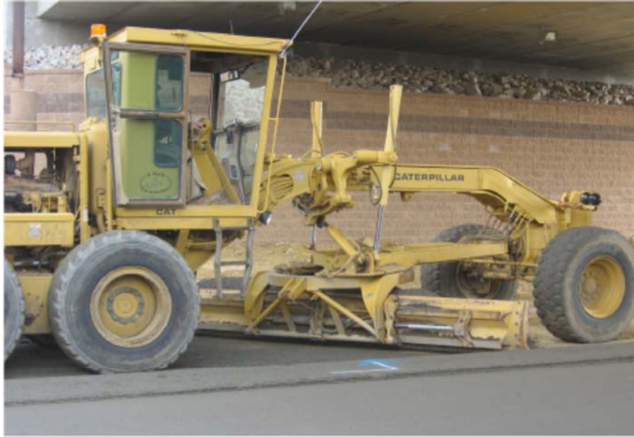
Fig. 1.3 A grader is used to prepare the base course
