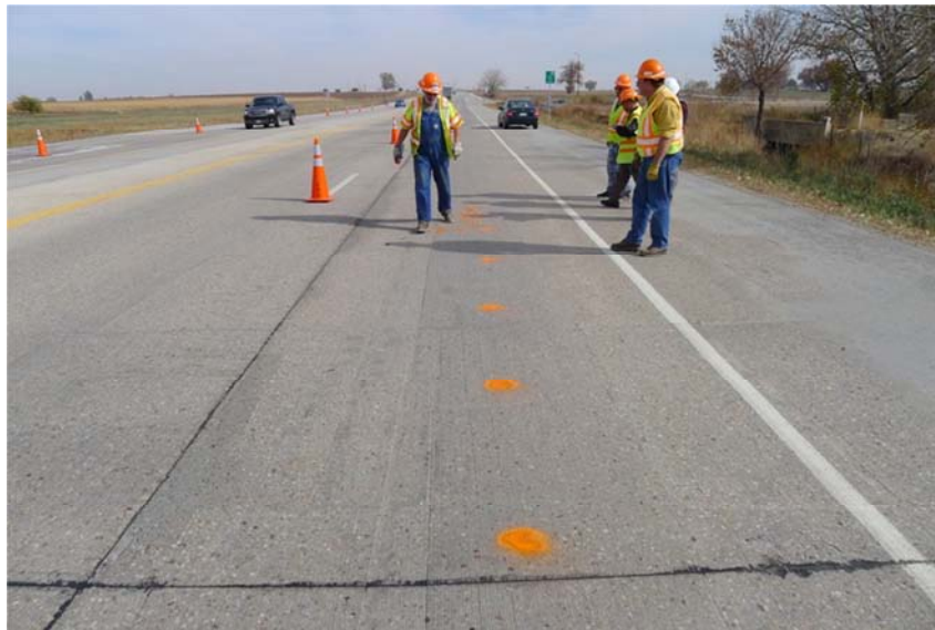
Fig. 3.15 Saw cut joints on the pavement at WB 66
