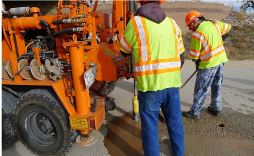
Fig. 3.20 Extracting concrete cores from the longitudinal middle strip at WCR 28
