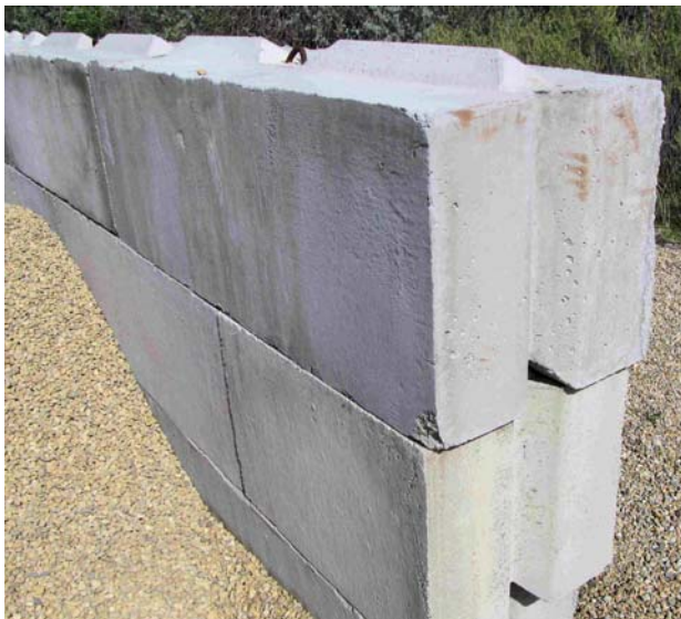
Figure 1. Stacked blocks form retaining wall. Note rebar hook in top middle.
