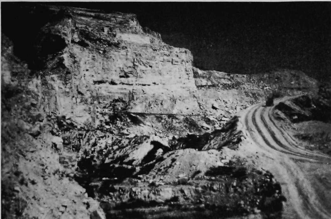
FIGURE 16 shows the working face at the Castle Concrete Co. limestone quarry near Colorado Springs. As in coal, the limestone extraction phase represents the greatest disturbance in the sequence of resource development. An active operation, whether it be a limestone quarry or the home kitchen during preparation of Sunday dinner, usually appears quite messy. Likewise, a limestone quarry--as the kitchen--can be, should be, and now usually is, cleaned up before the operation is finished.
