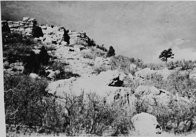
FIGURE 13. This rockfall occurred during a heavy rainstorm. The rocks rolled and bounded down onto an occupied building site in a platted subdivision.
