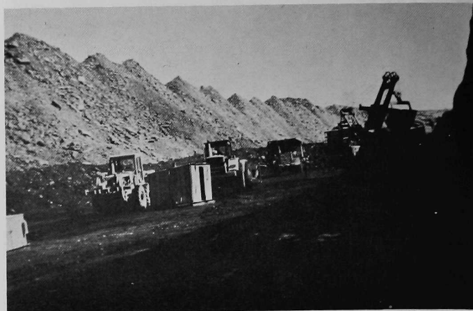
FIGURE 14. Extraction of the coal represents the most unsightly stage in the development process. The row of peaks to the left on the skyline is overburden deposited in the strip from which the coal has been removed in a previous pass. After the coal (foreground of this photo) is removed by power shovels and trucks, the next pass utilizes a dragline to move the overburden from the right to the void where this coal was removed, leaving another row of conical peaks. In the reclamation process, these peaks must be graded to a gently undulating surface to inhibit erosion and provide the base for revegetation. Care must be exercised that toxic materials are buried and not left at the surface. Normally, soil materials are stripped before overburden is removed and are placed on graded overburden from a previous strip. Plant species chosen for reclamation depend on climatic conditions, soil types and the desired final land-use objectives.
