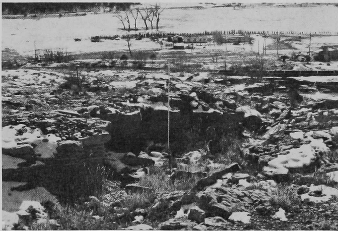
FIGURE 4. Collapse over room of Lewis No. 1 mine. Pit is about 10 ft by 15 ft and is 3 ft deep. From 5 to 10 ft of coal was extracted at a depth of approximately 50 ft. Flume carrying irrigation water in middle background must be periodically reset because underground mine fires in this area are causing continued subsidence.
