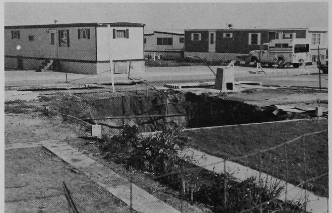
FIGURE 11. Subsidence pit at a trailer court in Lafayette. Ground began caving in the early morning of August 29, 1974, and continued to enlarge until noon. Final dimensions of the subsidence pit were 24 by 18 by 15 ft. The subsidence occurred in a vacant area, and only minor damage to utility lines was sustained. Had one of the large "mobile" homes shown in the background of this figure been parked on top of the subsidence area, it is doubtful that it could have been moved quickly enough to save it. This recent event is a dramatic example of continuing subsidence problems in an area where mining ceased over half a century ago.
