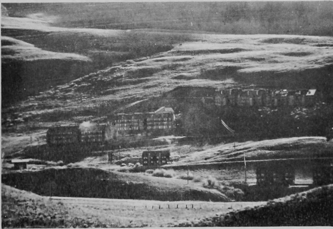
FIGURE 9. These condominiums are built on active earthflows.
