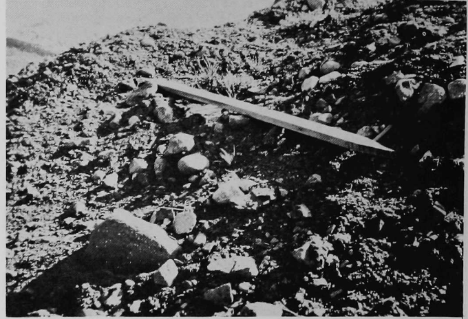
FIGURE 6. Close-up view of some typical unstable slope-forming materials. Lumber in photograph gives the approximate scale.
