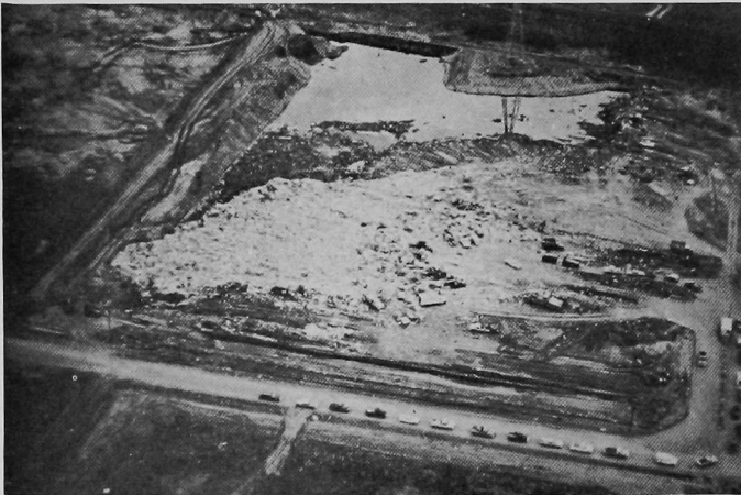
FIGURE 5. In the past, many abandoned gravel pits have been utilized as trash dumps. In many areas, ground water may become polluted and foundation conditions may cause problems for post-fill construction.
