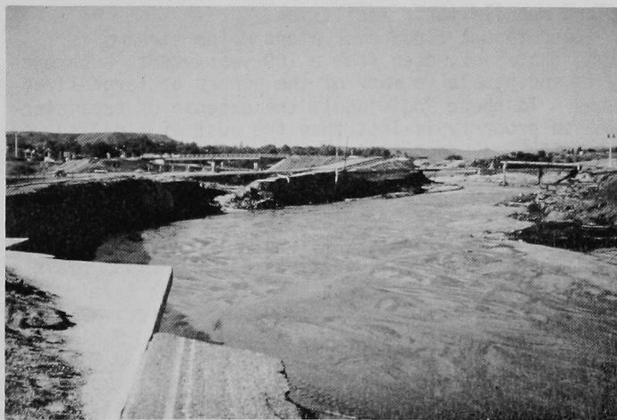
FIGURE 2. Washed-out service road adjacent to I-25 at Castle Rock as a result of 1965 flood. Note collapsed bridge in background.
