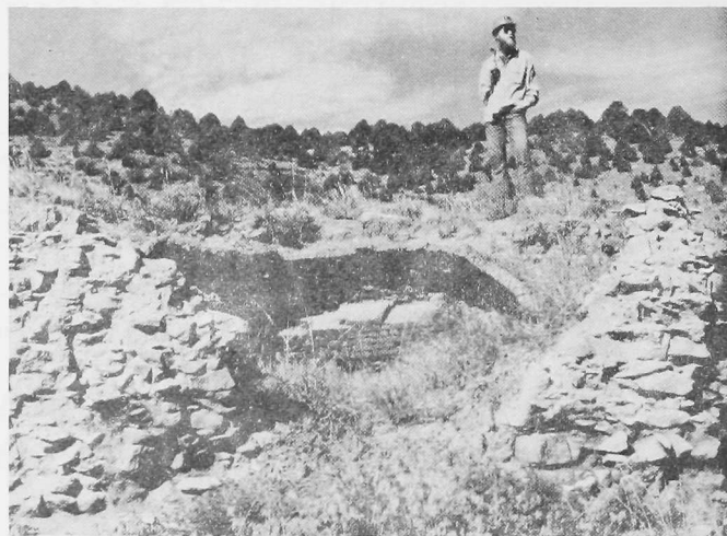
Figure 5. Ruins of a beehive coke oven located in the Raton Mesa coal region, near Ludlow, Las Animas County, Colorado.
