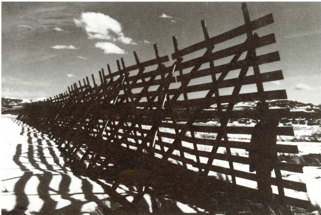
This Wyoming Design structure is 13.8 feet in height. With a porosity of 50 percent, it is very efficient in capturing and storing blowing snow.
