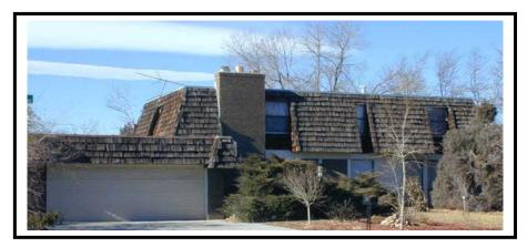
This Aurora fire station (upper left), home (left), and apartment house (lower right) are later examples that lack the double slope in the mansard roof. Instead, these Neo-Mansard examples rely upon a large pentlike projection below a flat roof to create the effect.
