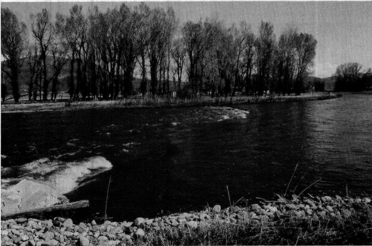
Angled rock structure across Elk River Photography by Jim Thornton, SCS, Denver, Colorado
