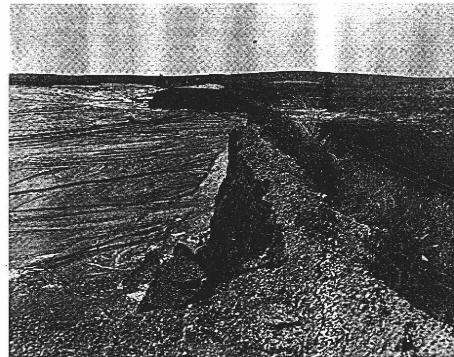
Jimmy Camp Creek and Marksheffel Road washout
