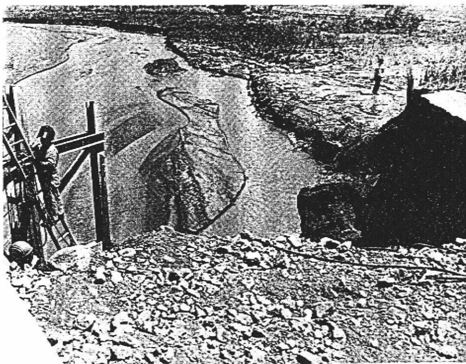
Bridge repair on Link Road and Jimmy Camp Creek .
