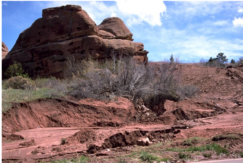
Figure 6 Example of erosion from urban development.
