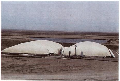
Photo 6. Digester Lagoon and Evaporative Lagoon at Colorado Pork.
