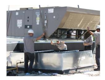
The upgrades to the City of Lafayette's facilities included new energy efficient roof top units for heating and cooling
