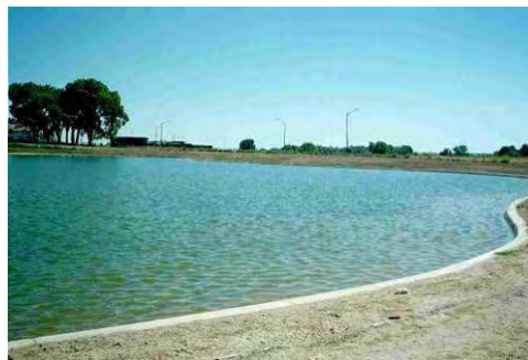
Fossil Ridge High School constructed pond allows on-site stormwater runoff to be detained for irrigation
