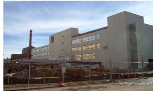
Colorado Department of Labor and Employment Silt fence minimizes construction disturbance
