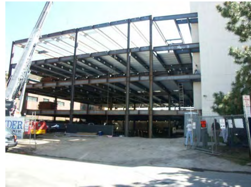
Colorado Department of Labor & Employment structural steel has recycled content and was manufactured locally
