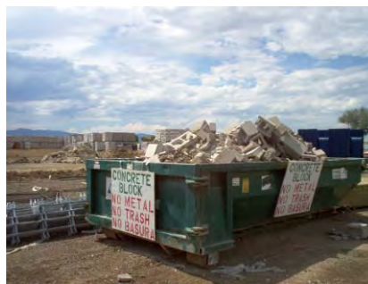
Poudre School District staggers recycling containers to save space on jobsites.
