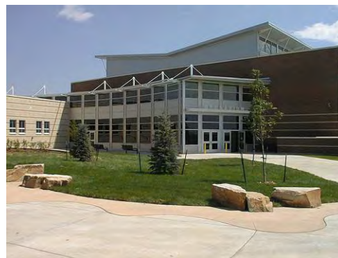
Fossil Ridge High School uses concrete and trees to minimize heat island Courtesy: RB+B Architects
