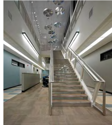
Colorado Springs Utilities Laboratory uses high-efficiency lighting with diffusers, automated dimming, photo sensors, and interior windows that provide shared lighting. Courtesy: Ed LaCasse Photography
