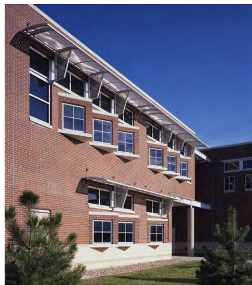
Fossil Ridge High School uses details such as tilting windows in a west wall to minimize summer overheating.
