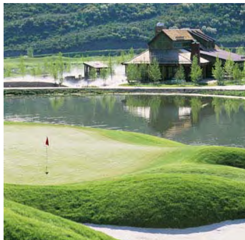
Snowmass Golf Clubhouse uses the pond on Hole 18 of the golf course as a heat sink for water-source heat pumps in summer and winter, shown under construction (top) and completed (bottom). Courtesy: Aspen Skiing Company
