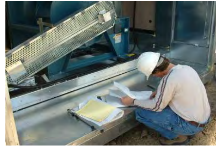
Commissioning Field Work
