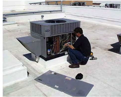
Commissioning Field Work
