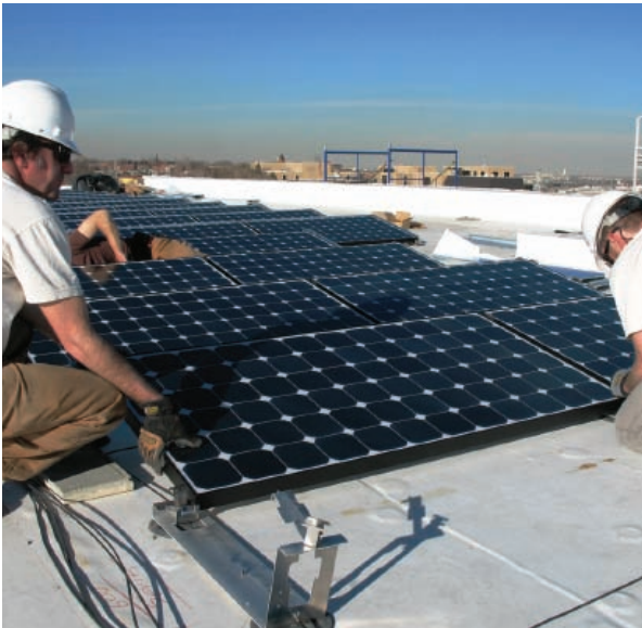
Left: Employees of Boulder-based Namaste Solar Electric install a photovoltaic system at the River Clay Condos in Denver; Right: A worker installs Johns Manville blown-in fiberglass insulation to improve the energy efficiency of a new home.
