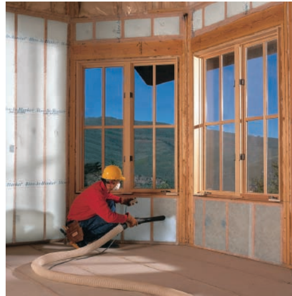
Left: Employees of Boulder-based Namaste Solar Electric install a photovoltaic system at the River Clay Condos in Denver; Right: A worker installs Johns Manville blown-in fiberglass insulation to improve the energy efficiency of a new home.
