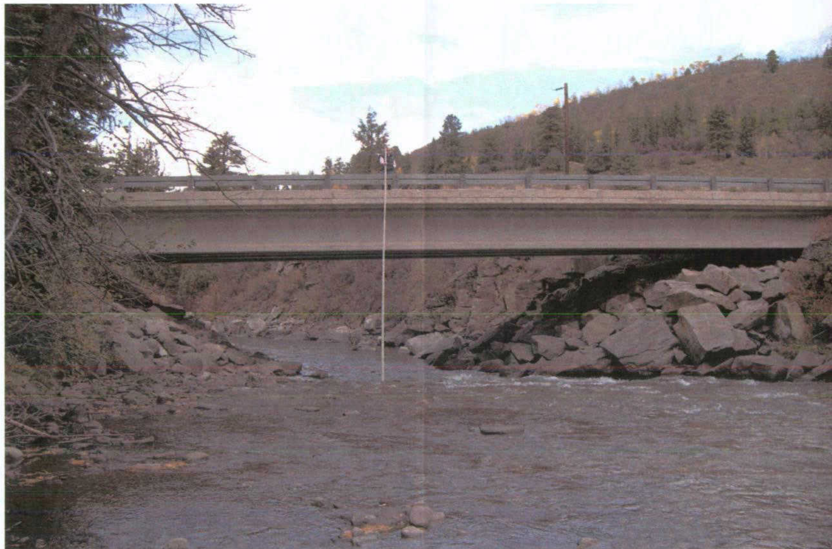
Prospect Ranch Bridge (County Road 3): Upstream Looking Downstream
