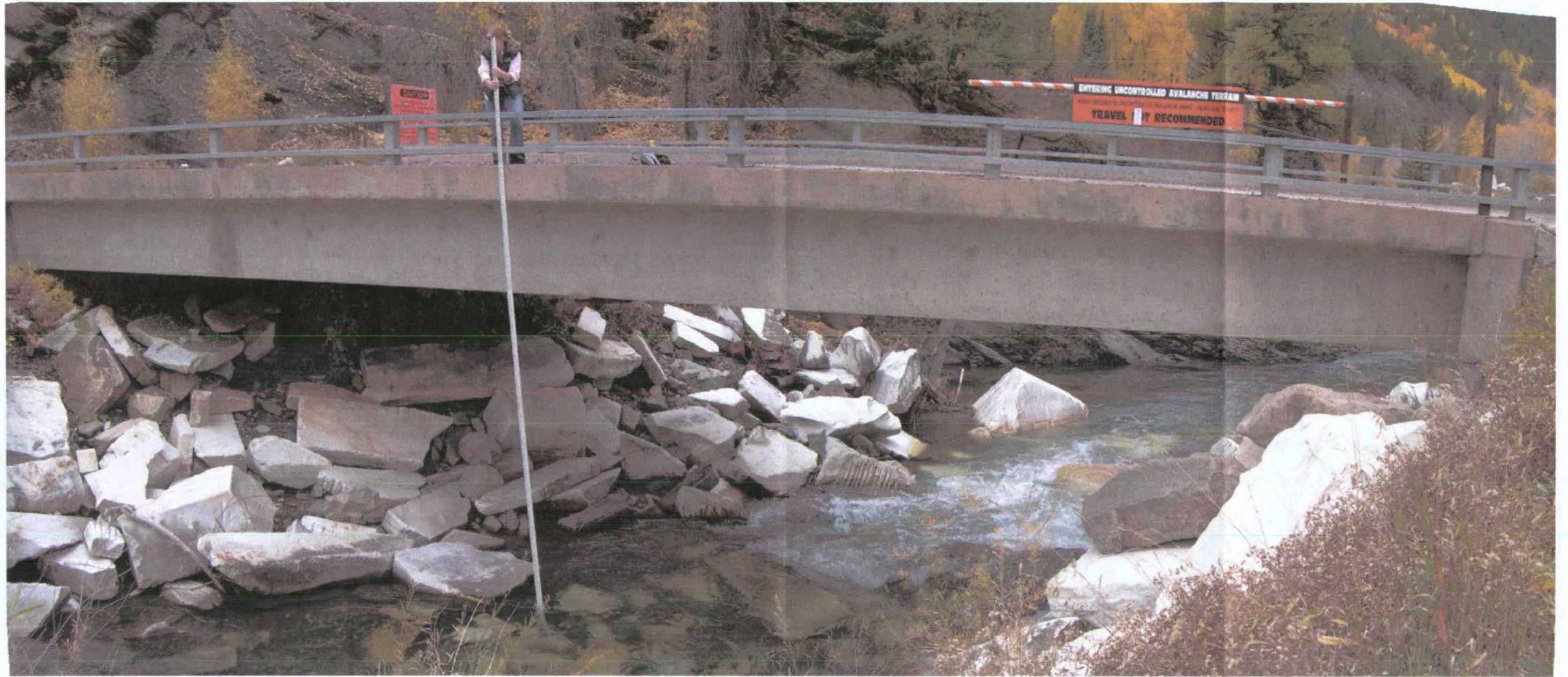
Town of Marble Bridge (Highway 30): (Upstream Looking Downstream)
