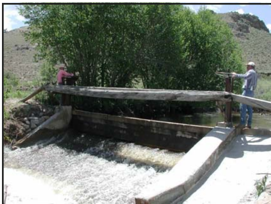
Arch Ditch Diversion Structure
