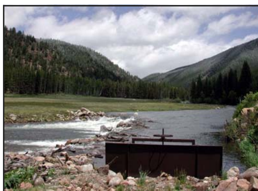
Diversion Structure on Crystal Creek
