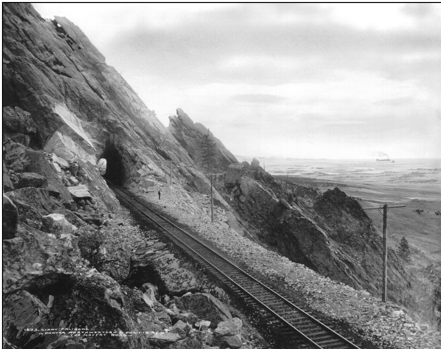
Tilted layers of 300-million year old Fountain Formation sandstone along the old Moffat Road. These sedimentary rocks were originally flat; they were uplifted into their present position when the Rocky Mountains were formed about 65 million years ago. (Photograph by L.C. McClure, 1904. Courtesy Denver Public Library Western History Department)
