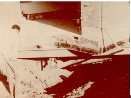
Figure 27a. Subsidence pit under the corner of a house. The beam, drilled pier and jack hold the house in position and level the building.
