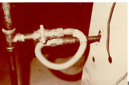
Figure 26a. Flexible gas coupling.
