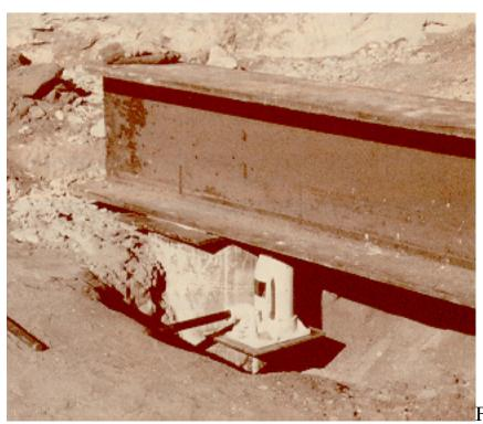
Figure 27b. Close up of a beam, drilled pier and
