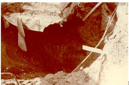
Figure 21. A subsidence pit under the corner of a house. Note the utility being held up by string. (*photo courtesy of L. Floyd Office of Surface Mining*)
