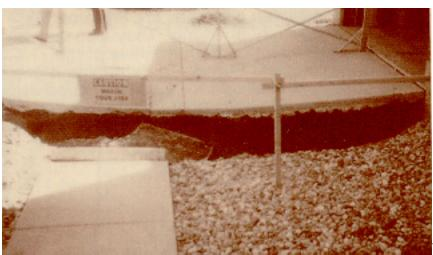
Figure 18. Mine shaft fill collapsed under this
