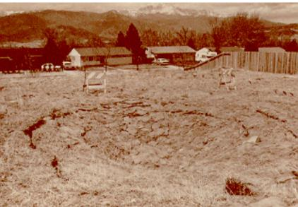
Figure 12. A subsidence trough in a vacant lot. Tension cracks are visible around the sag. (*Colorado Mined Land Reclamation Division*)
