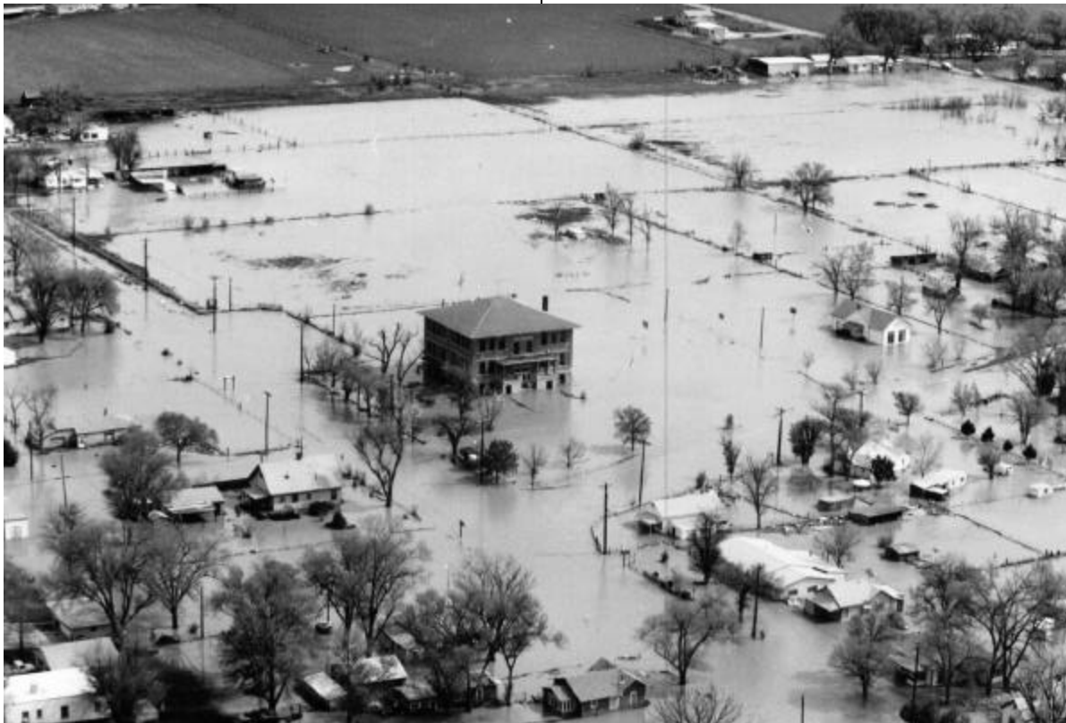
May 1999 Flooding in Otero County, Colorado - La Junta Middle School, Built in 1901, on the State Historic Registry.
