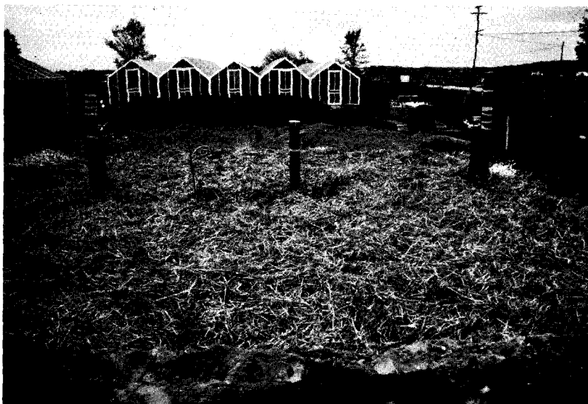
Fig. 9. Place 3 to 4 in. of straw or marsh hay (uncompacted) on top of stones.
