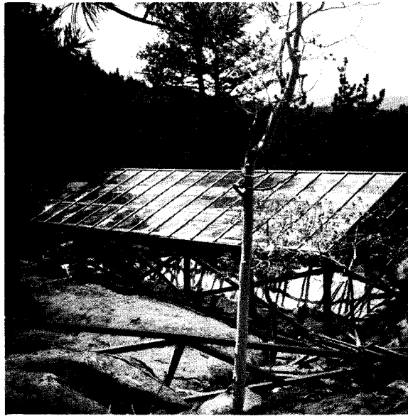
Figure 11. Full Scale Unit During Construction.
