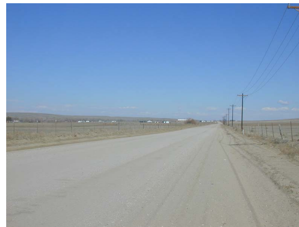
Figure 13-3--Kiowa-Bennett Road in Elbert County
