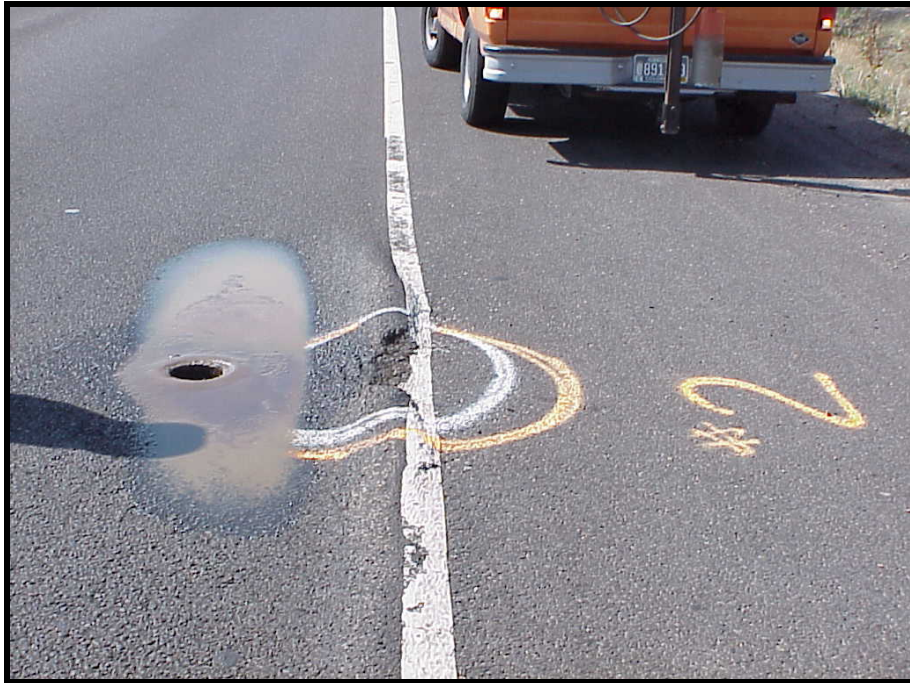
Figure 27: Coring location 4 illustrating quarter inch ruts in the number 2 lane
