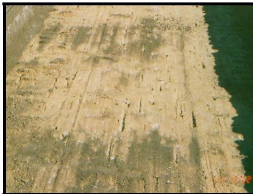
Figure 3: Roadbase exposed during asphalt remediation
