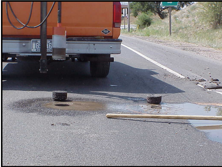
One to two inch ruts in the number 2 lane where truck traffic was concentrated
