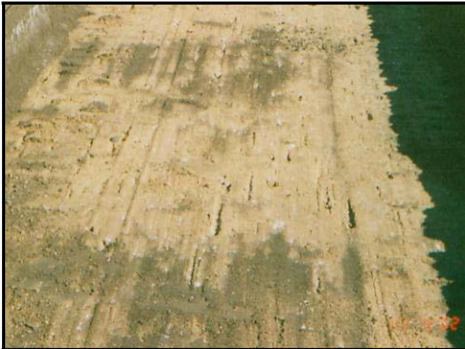
Figure 30: Roadbase exposed during remediation
