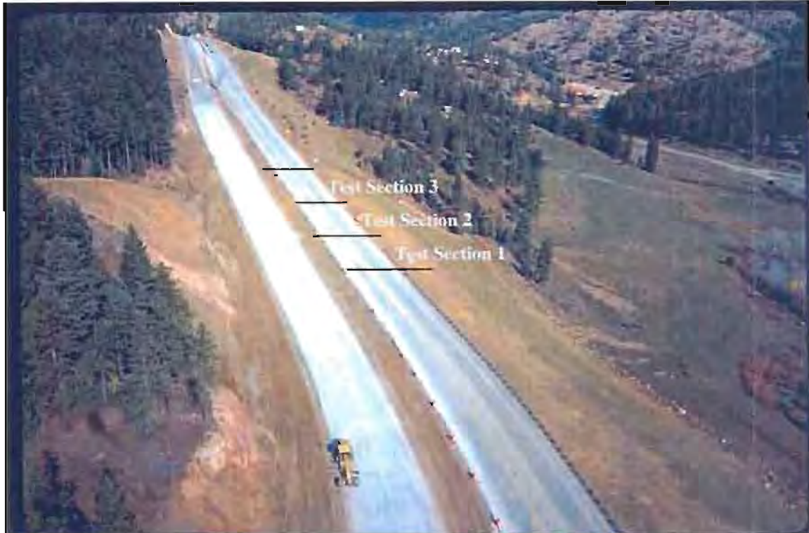
Figure 2. Oblique view looking east at Test Sections 1 through 3 along US285.
