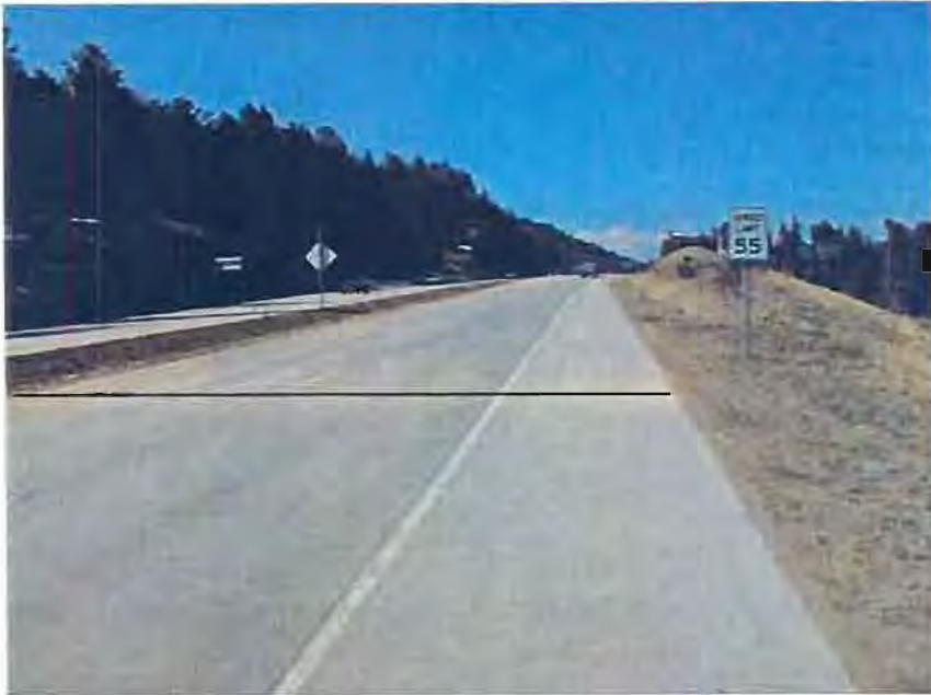
Figure 3. View looking east at transverse tining Test Sections 1, 2 and 3 along US285 mileposts 244.42 to 224.53.
