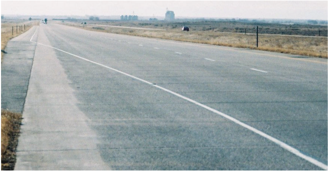
Figure B-9. Good Pavement Condition on I-76 (Eastern Site).
