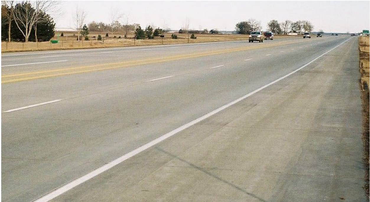
Figure B-13. Good Pavement Condition on US-34.
