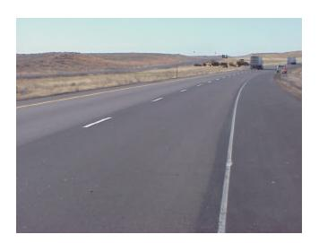
Figure 11. This photograph was taken 4 years after construction. There are two areas where segregation has began to appear.
