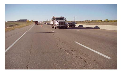
Figure 1. Longitudinal cracking was found on this project as shown in this photograph. This cracking pattern was consistent throughout the entire length of the project.
