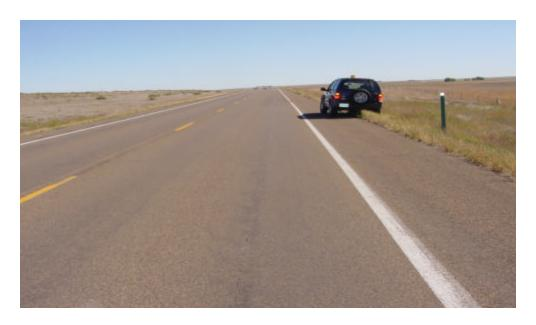
Figure 14. This distress was a reflective crack. Note the linear straightness and low severity of the crack.
