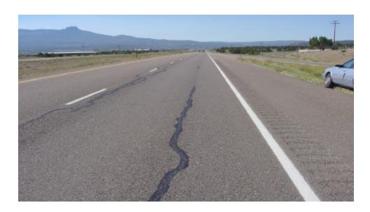
Figure 15. This crack was top-down. Although the crack is straight, the severity was enough to warrant crack sealing.
