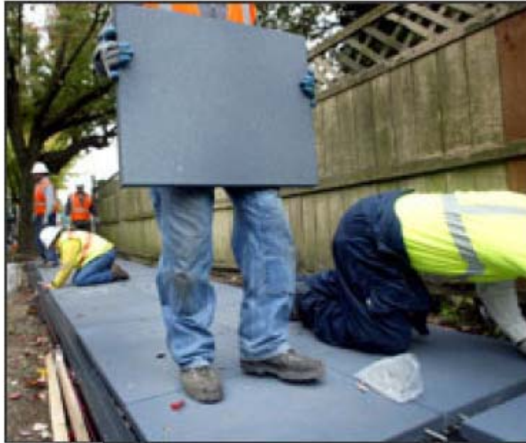
Figure F-4 Rubber Sidewalk Installation
