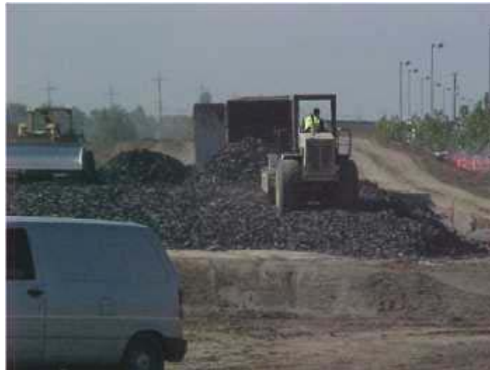
Caltrans uses shredded tires in highway embankments
