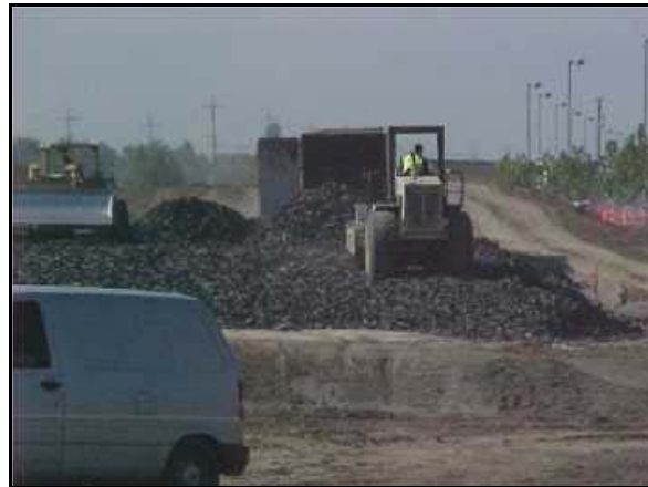
Figure 4. Caltrans Uses Shredded Tires in Highway Embankments
