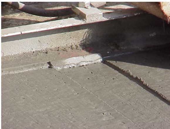
Figure 2. Small pieces of steel welded to the screed formed the grooves.
