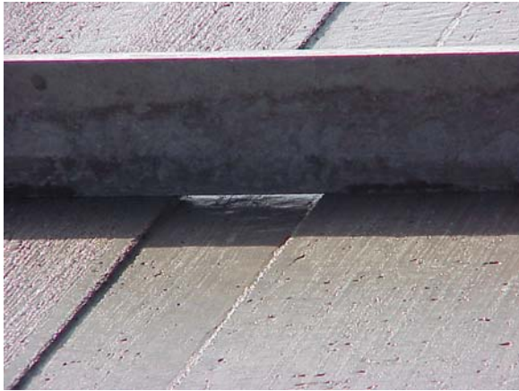
Figure 1. Shoulder stripe groove formed in plastic concrete.
