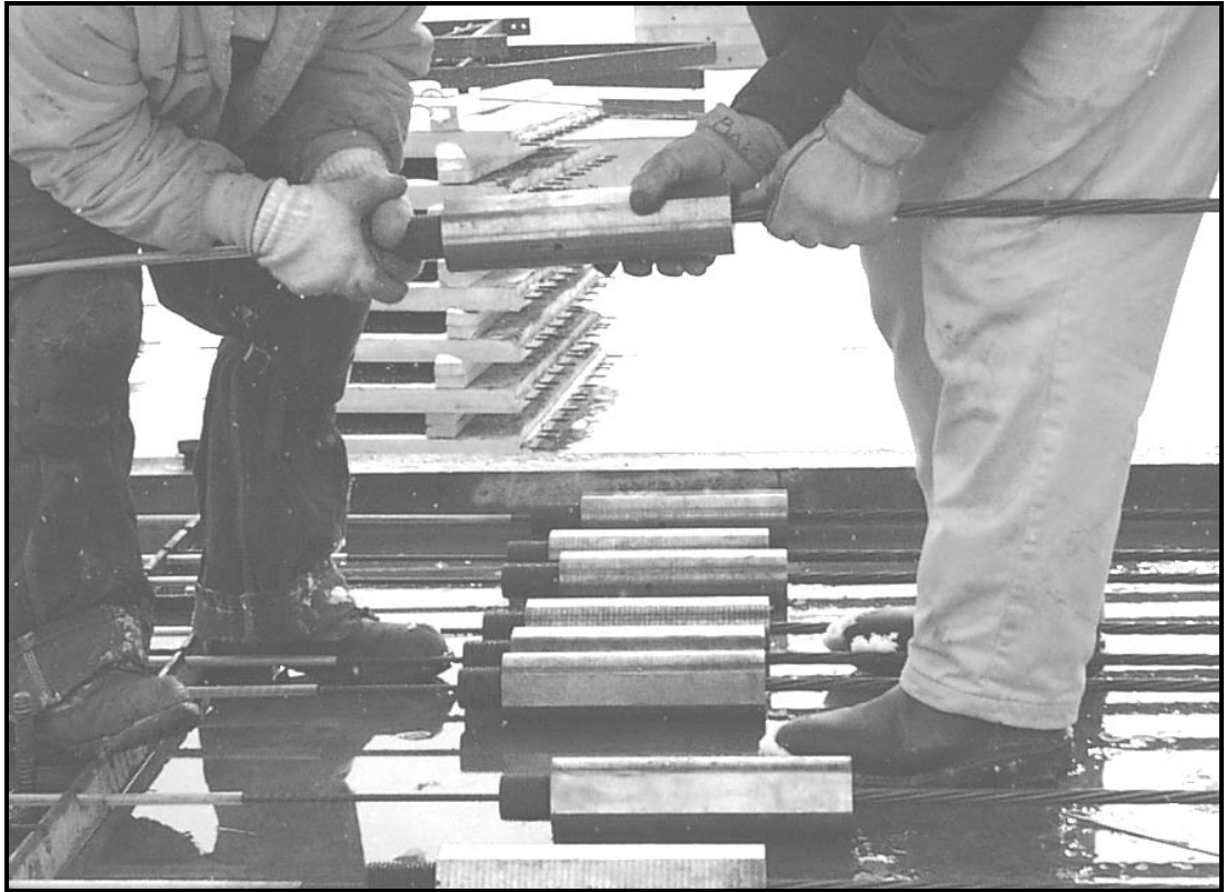
Figure 4.4 Coupler application
