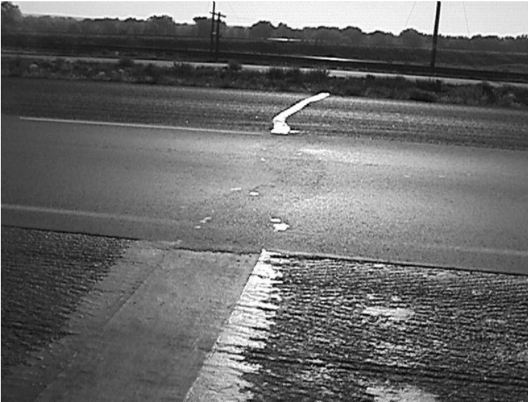
Figure 13 –Typical Petrotac treatment after the trenched section has been overlaid.
