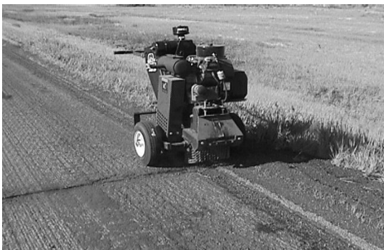
Figure 10 – Equipment used to rout the crack prior to filling it with sealant.
