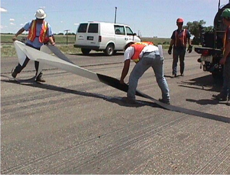
Figure 7 – Petrotac placement.
