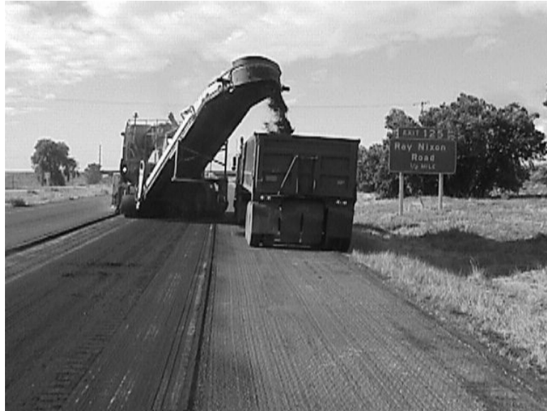
Figure 2 - Rotomilling operation.
