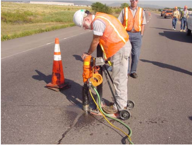
Figure 16 - Coring operation on the affected joint.
