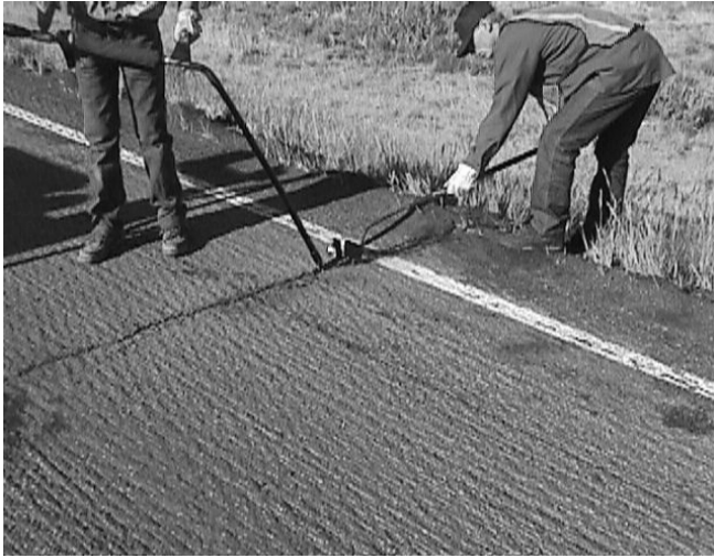
Figure 11 – Filling the crack with crack sealant.
