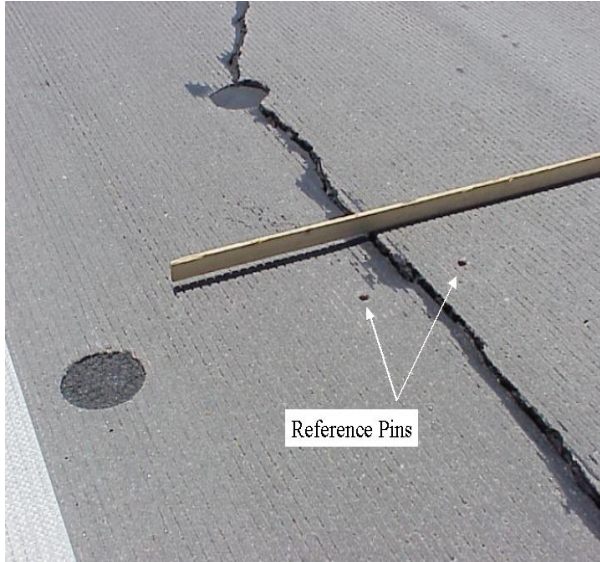
Figure 26: Differential Settlement
