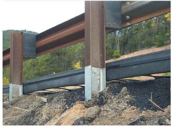
Figure 24. Inadequate base for the DFC.
