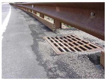
Figure 19. A hollow section of composite lumber curb ends at a drain.
