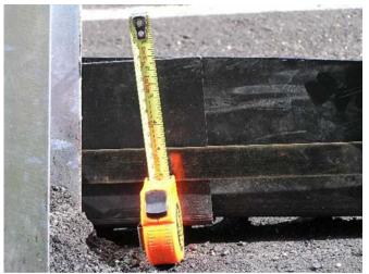
Figure 11. Air gaps between the curb material and the pavement surface.
