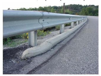
Figure 2. Extruded curb - concrete in this case.
