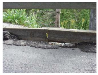
Figure 3. Wood curb can twist and warp.
