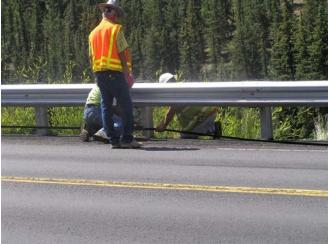
Figure 12. Wavy curb face between guardrail posts is mainly a cosmetic problem.
