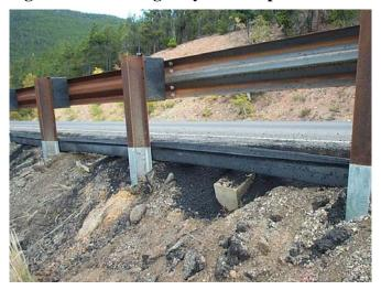
Figure 23. Slopes start under the guardrail.
