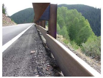
Figure 20. A small movement of the guardrail separated this curb from the pavement.
