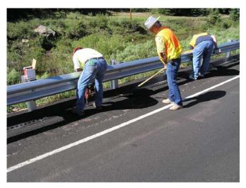
Figure 10. Holding DFC tight against the post base and the pavement with a shovel.
