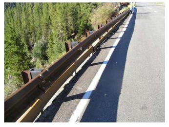
Figure 7. Slight movement of the guardrail can render the curb completely ineffective.
