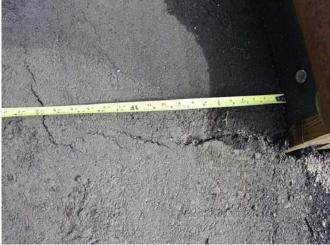
Figure 14. Cracks along the edge of the HDPE Figure 15. Cracks are developing at the end and on US-24.
