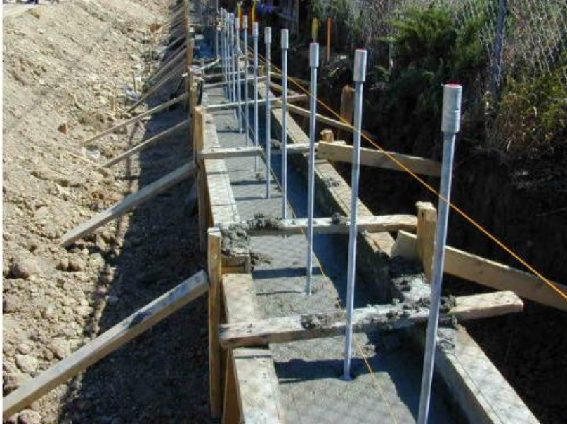
Figure 4. Photograph of grade beam with tendon anchorages installed.
