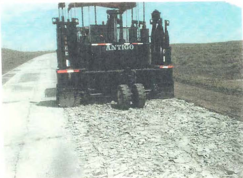
Figure 6. Multi-head Hammer
