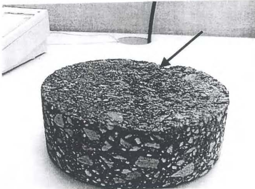
Figure 9. Core of Top-Down Cracking, 9/16/2001.
