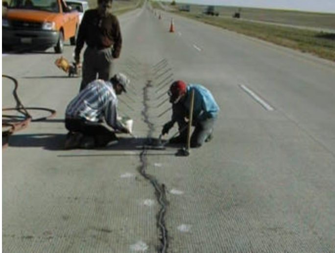
Figure 4. Installation of stitches on I-70 at Agate.
