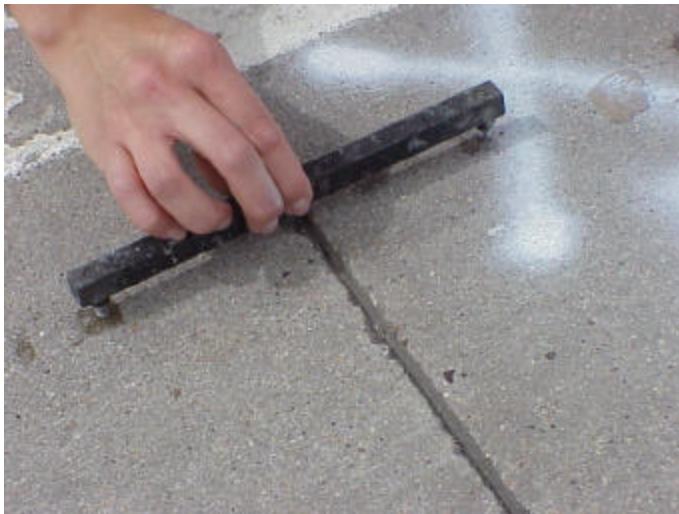
Figure 3. Reference pins installed across a joint.
