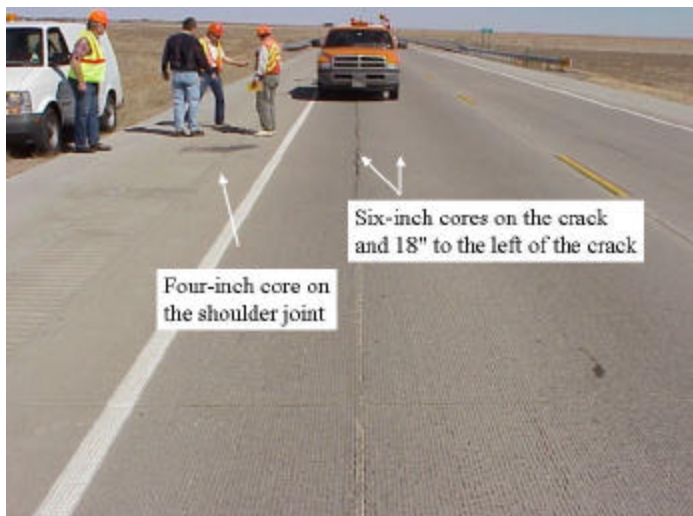
Figure 5. Core locations on the vibrator trail - US-287 southbound.
