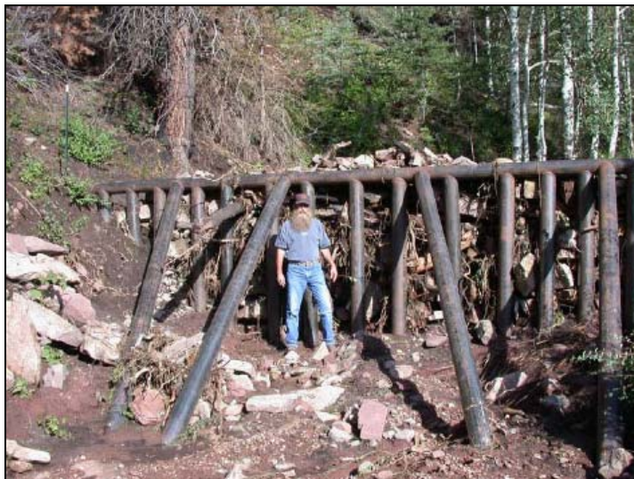
Figure 4 – A debris rack above Lemon Dam (near Durango, CO) successfully contained coarse material from a debris flow after the Missionary Ridge Fire of 2002 (from Florida Water Conservation District, 2003).
