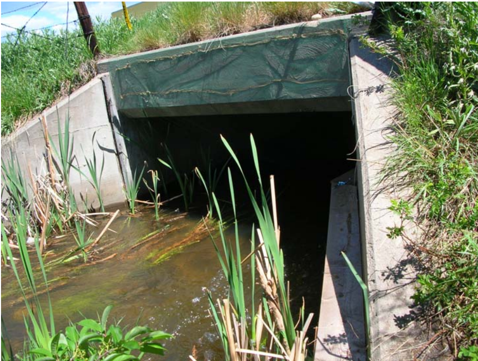
Culvert 2. Marshallville at U.S. 36.
