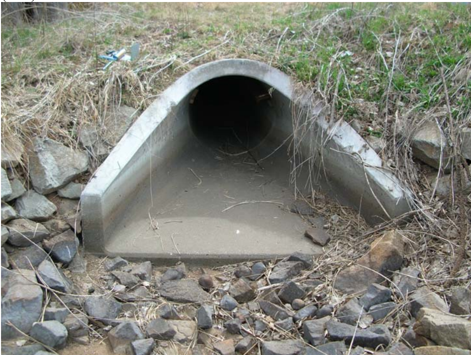
Culvert 4. East Boulder Ditch. This is a round concrete culvert and the smallest diameter (1 m) of all the culverts.
