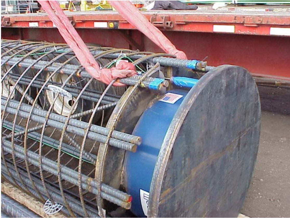
Figure 4.1. Photo of the O-Cell Placed in the Broadway Test Shaft.
