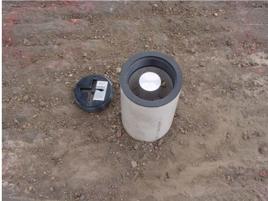
Figure D.5. Reference Rod Assembly Installation
