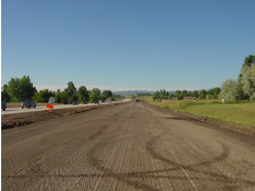
Figure C.1. Milled Surface of Existing Asphalt Pavement
