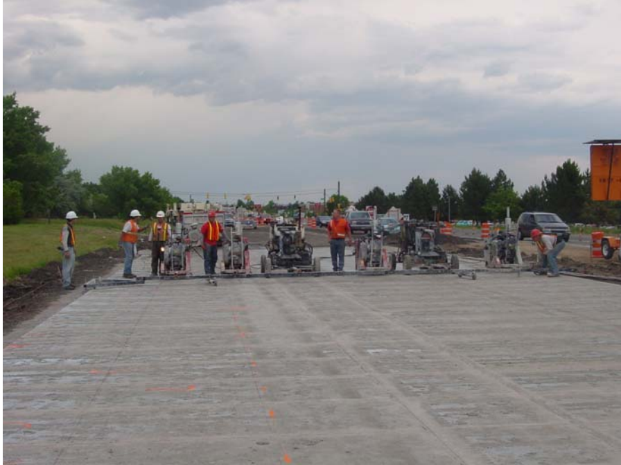
Figure C.4. Sawing Longitudinal Control Joints
