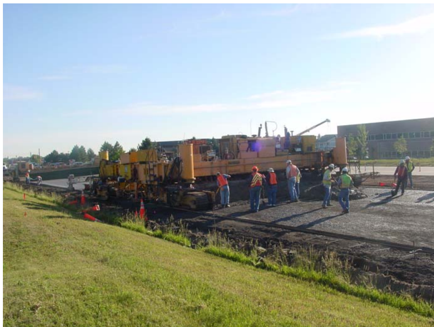
Figure C.2. General View of the Thin Whitetopping Paving Operation
