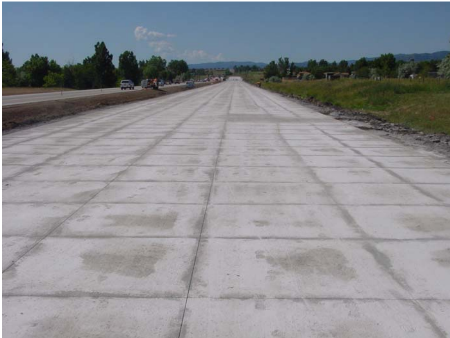
Figure C.5. Pavement Surface After Joint Sawing
