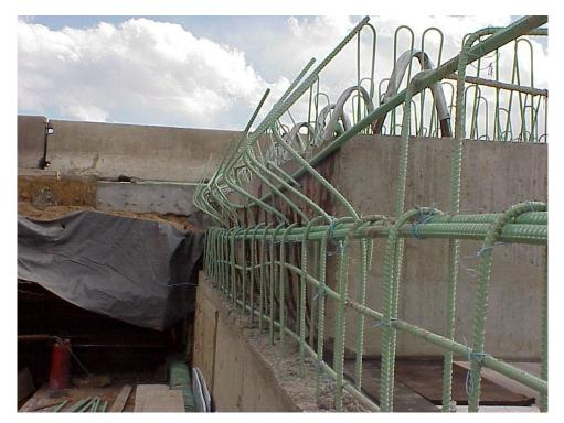
Figure B-33. Abutment wall and some girders. The stage that follows is pouring the concrete for the bridge deck and the rest of the abutment wall and girders. The overlapping steel from girders, abutment wall, and bridge deck will strongly attach the bridge superstructure to the abutment wall without any joint (integral abutment).
