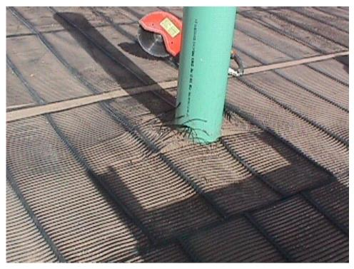
Figure B-24. The geogrid was cut to fit over a drain pipe that went down through the middle of the structure. The pieces of geogrid were offset from one layer to the next so the longitudinal joints did not line up vertically.
