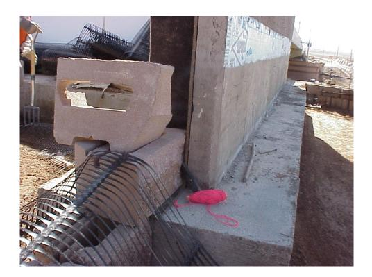
Figure B-38. The edge of the wing wall and upper MSE wall. Expansion joint material was placed between blocks and leveling pad and between blocks and the wing walls.
