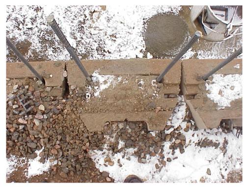
Figure B-27. The top two rows of blocks were filled with concrete. Steel rebars inserted in the plastic concrete were later bent over to tie the concrete cap at the top of the front MSE wall.
