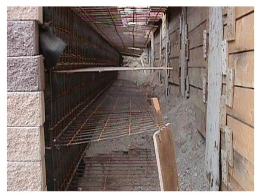
Figure B-19. Temporary wire mesh facing was used to support the northern face of the Phase I structure until the Phase II structure was built and tied to the Phase I structure. The backfill in between the wire mesh reinforcement was contained using wrapped fabric that also facilitated backfill drainage. To the right is a closer look at the shoring supporting the old bridge structure.
