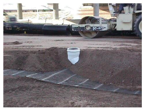
Figure B-23. A vertical drain pipe was installed inside the MSE Walls.
