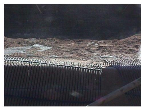
Figure B-16. Around the corners of the lower MSE walls, where geogrid from the front and side of the structure overlapped, a thin layer of fill material was placed between these geogrid layers to provide friction between them.
